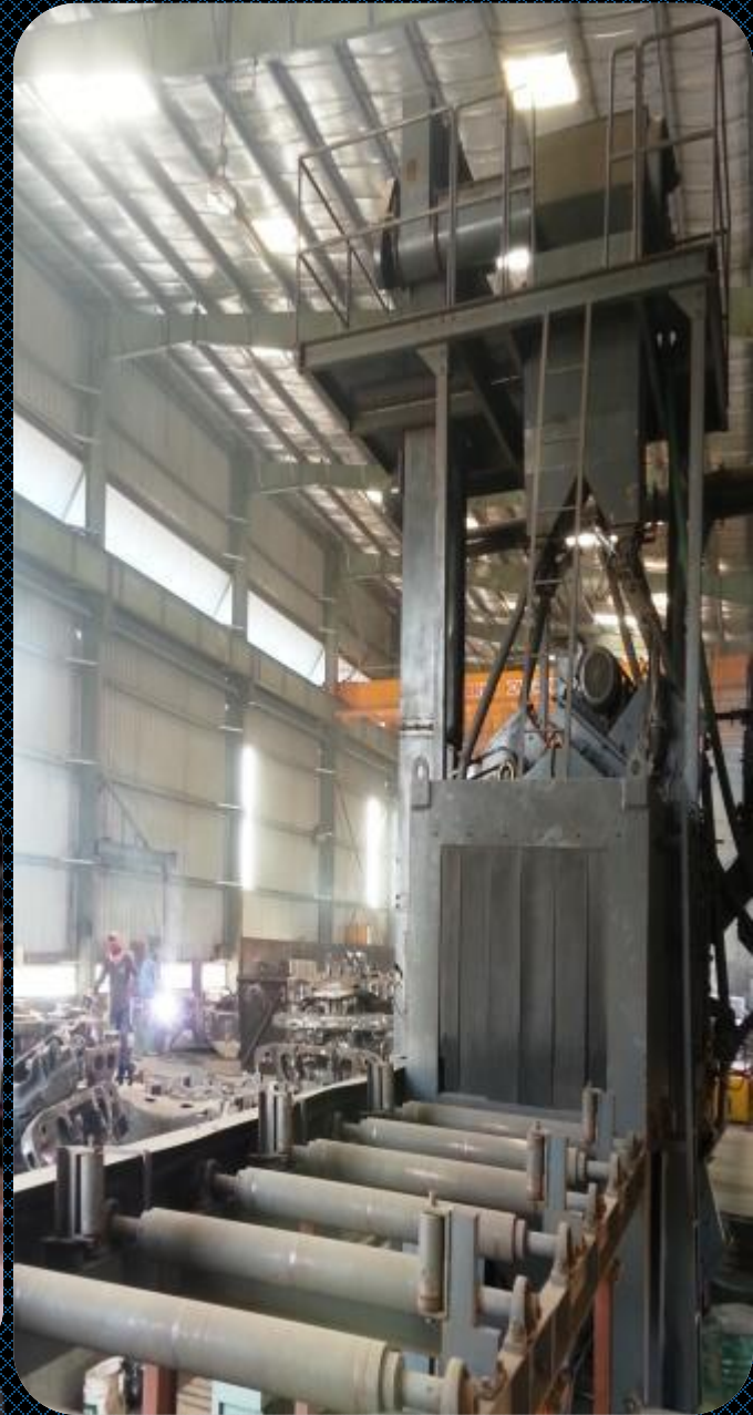
Shot blasting Facilities
