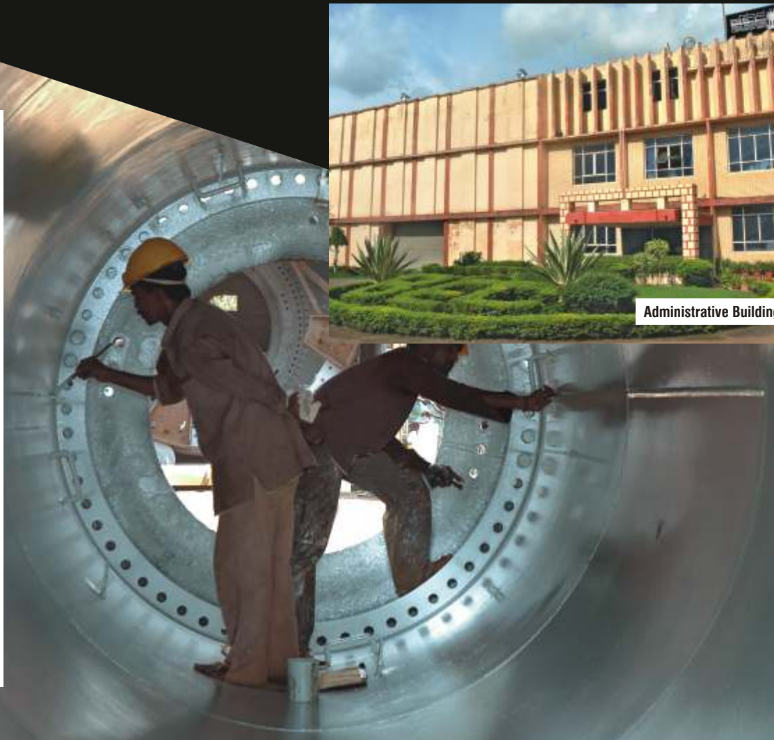
Wind Mill Tower - Under Painting
